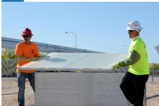
4 Position into bracket "T"
