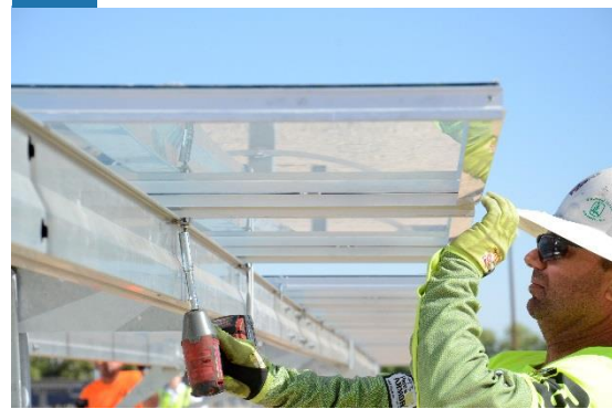
6 Secure bracket bolt
