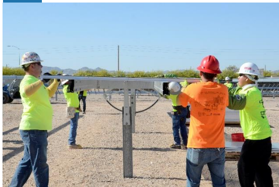
4 Position into bracket "T"
