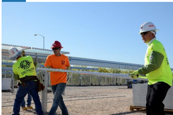
5 Align in the bracket "T"
