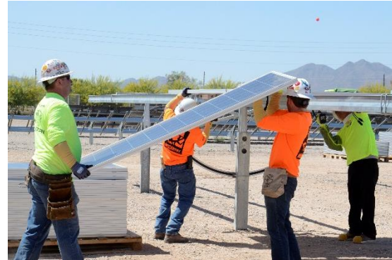
c-Si install on Exosun Structure
