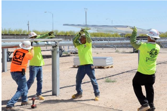
S6 install on ATI Structure
