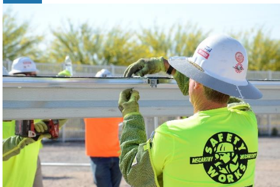
5 Align in the bracket "T"
